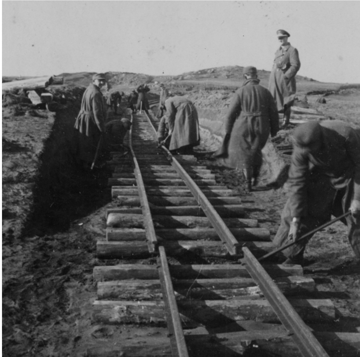
From the construction of Lundebanen at Lista. This narrow-gauge railway was built to transport supplies and building materials from the harbour in Lundevågen to the German construction sites at Lista. In addition to the airfield, the batteries in Marka and at Tjørveneset were the biggest sites. The railway had several side-tracks, for example to the sand washing plant at Nesheim and the quarry in Mabergåsen. Photo illustration, not pertaining to the individuals described in this story. PHOTO: LISTA MUSEUM
